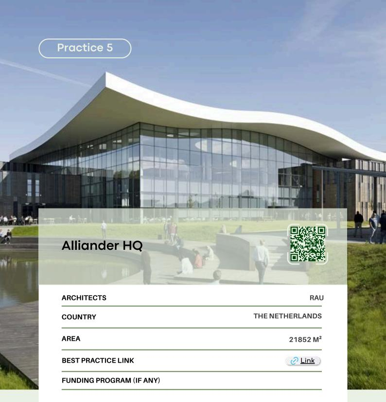
Alliander's Duiven office campus was sustainably renovated under circular-economy principles by retaining six blocks and linking them with a new atrium. Roughly 80% of materials—ceiling panels, doors, plumbing fixtures—were reused on-site or repurposed elsewhere, cutting waste and curbing new resource use. The project achieved BREEAM Outstanding certification.
