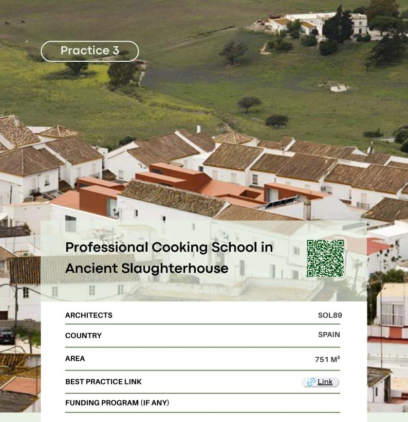
Sol89 converted a 19th-century slaughterhouse in Medina Sidonia into a cooking school, retaining its whitewashed walls, stone and brickwork, and Phoenician columns under a unifying ceramic roof. The original courtyard layout persists alongside new patios for ventilation and herb gardens, while concrete slabs with wooden formwork reinterpret local building methods to blend history and modern function.
